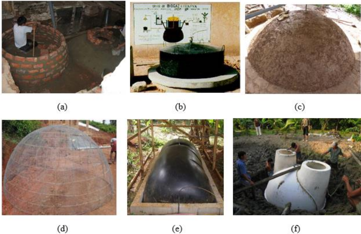
84 85 Figure 1: Applications of the six most common biogas digesters: (a) fixed dome 1 ; (b) floating 86 drum 2 ; (c) earth-pit 3 ; (d) ferro-cement cage 4 ; (e) balloon 5 ; and (f) composite material 5 .
