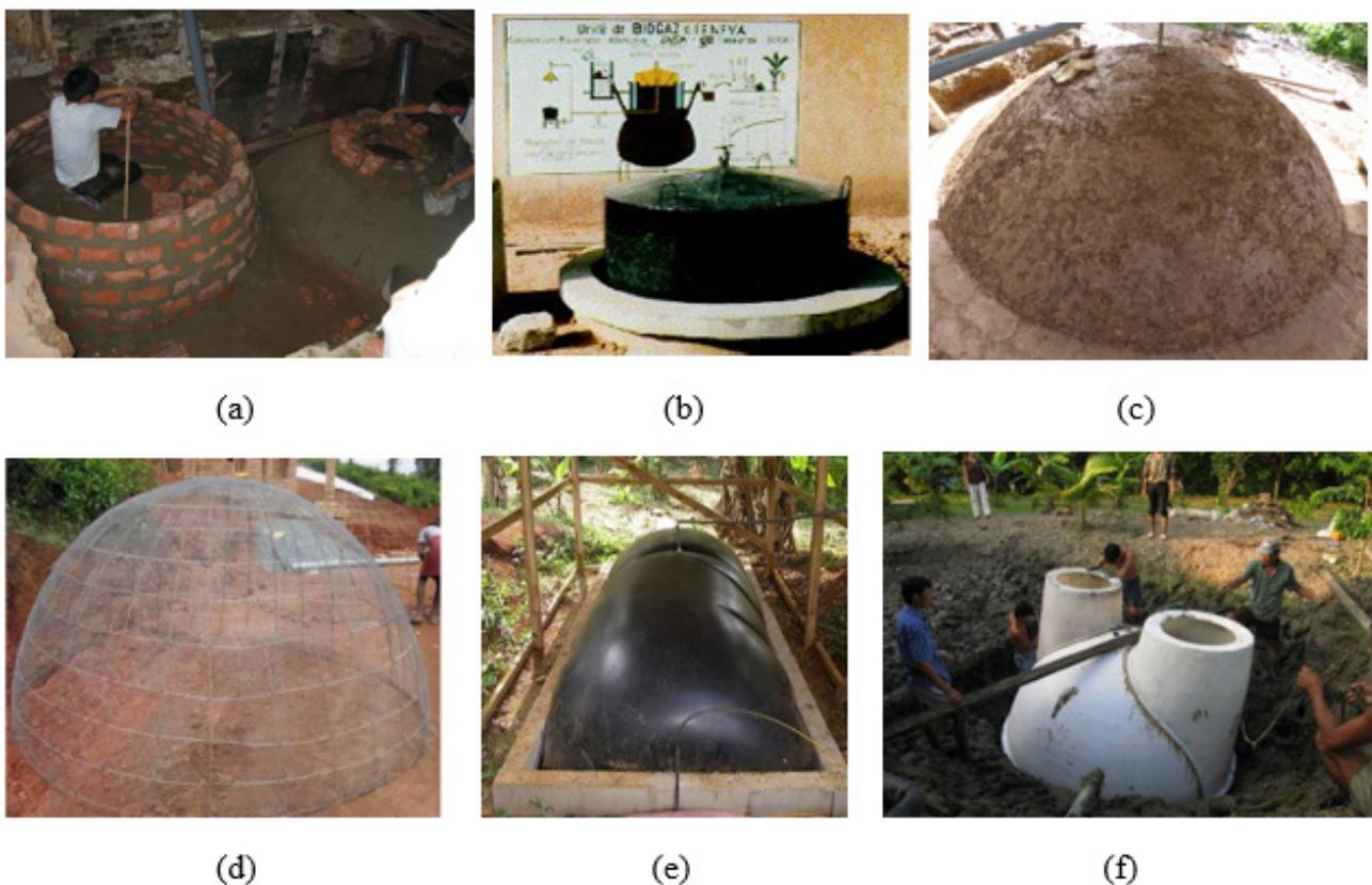
Figure 2: Applications of the six most common biogas digesters: (a) fixed dome<sup>1</sup>; (b) floating drum<sup>2</sup>; (c) earth-pit<sup>3</sup>; (d) ferro-cement cage<sup>4</sup>; (e) balloon<sup>5</sup>; and (f) composite material<sup>5</sup>.
