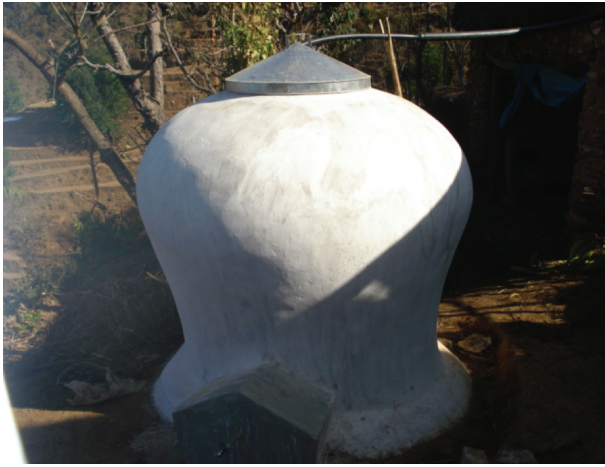
Figure 1: 6500 L RWHS installed by NEWAH.
