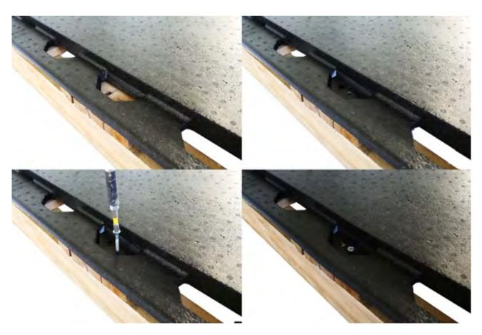
Figure 2: Installation of an Emergency Floor tile onto a wooden shipping pallet
