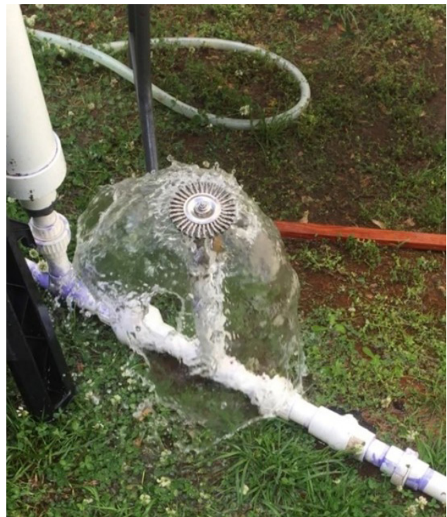
Figure 3: The operating test ram pump
