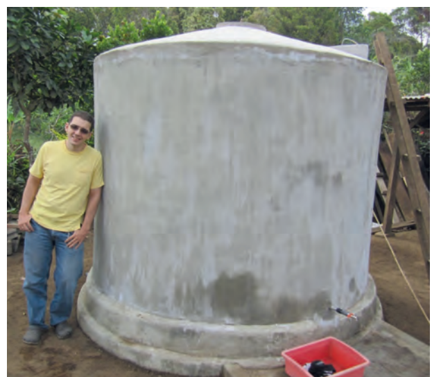
Figure 7: Example of a storage tank.
