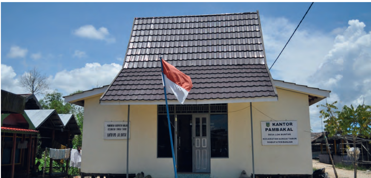
Figure 9: Example of roofing – village office.
