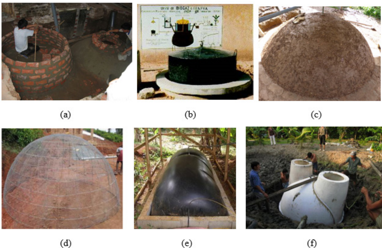
Figure 2: Applications of the six most common biogas digesters: (a) fixed dome 1 ; (b) floating drum 2 ; (c) earth-pit 3 ; (d) ferro-cement cage 4 ; (e) balloon 5 ; and (f) composite material 5 .
