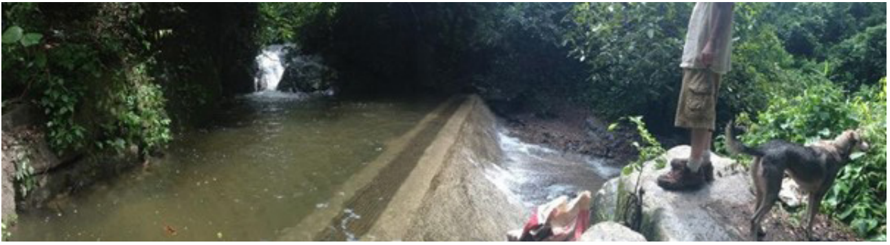
Figure 1: Catchment structure with water overflow during the end of the rainy season (dog and person included for scale)
