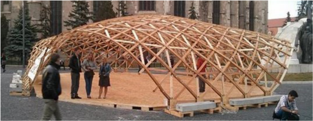
Figure 1: ZA Pavilion, fully constructed in Cluj, Romania (Photo by Dragos Naicu)
